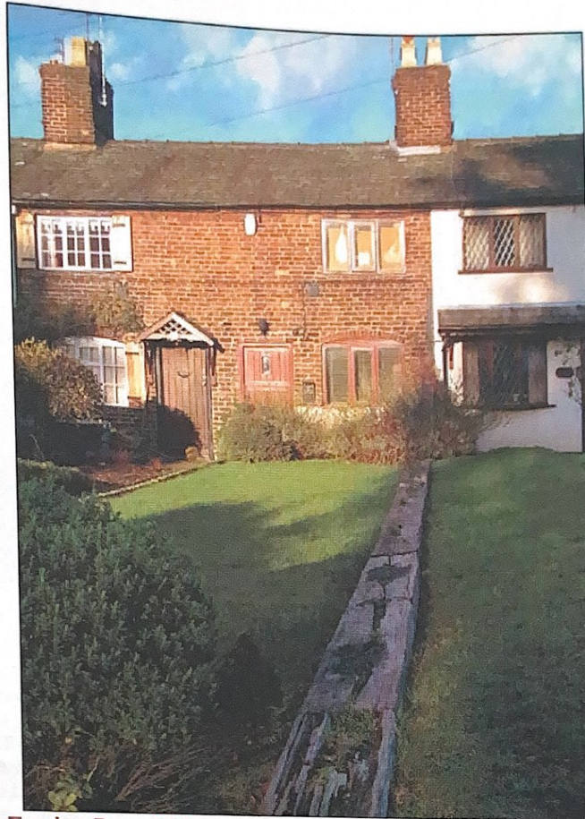
at Twelve Row, Kidsgrove sleepers form the house boundary
