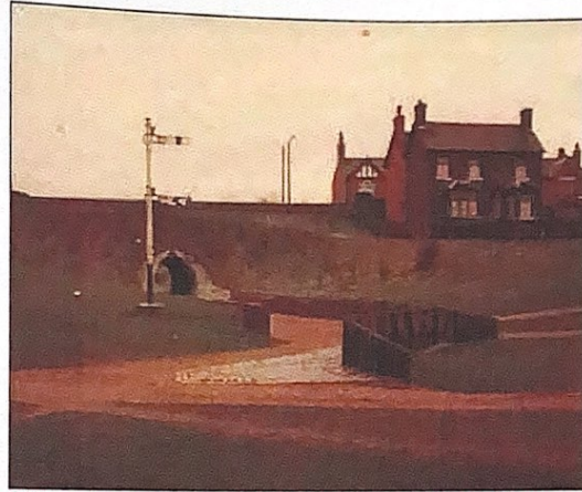
view of the site of the disused Tunstall Railway Station now converted into a Greenway.
